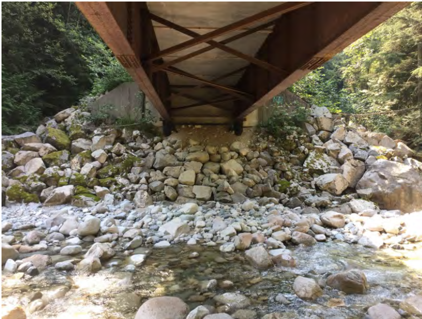
Left Bank Abutment when facing downstream
