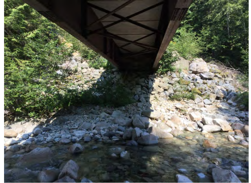
Right Bank Abutment when facing downstream
